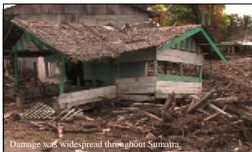
Damage was widespread throughout Sumatra.
